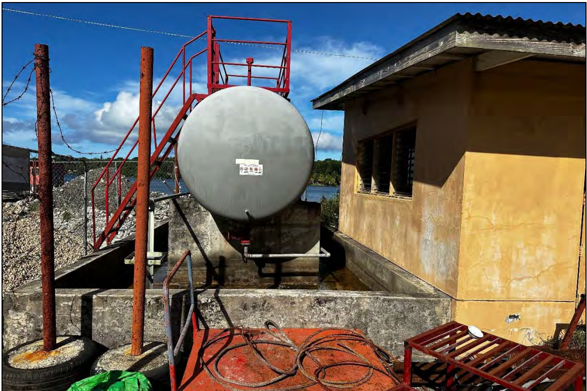
Photo 16: Overview of 10,000-liter diesel AST located at the YFA facility. Note: A concrete containment basin sits beneath the AST. Photo is looking south.
